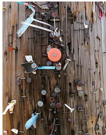
Despite the safety gear worn by linemen to avoid contact with rough surfaces, objects used to attach signs to poles can poke through gloves, boots, and protective clothing and cut the linemen.
